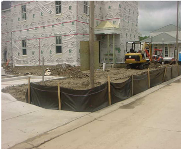
Silt fencing used as a sediment barrier.
