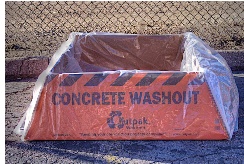
Properly installed concrete washout.
