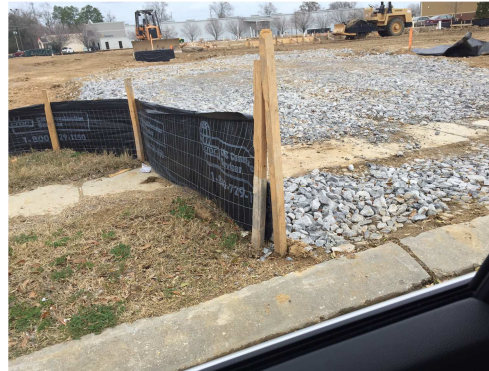
Properly installed silt fence and construction site entrance.
