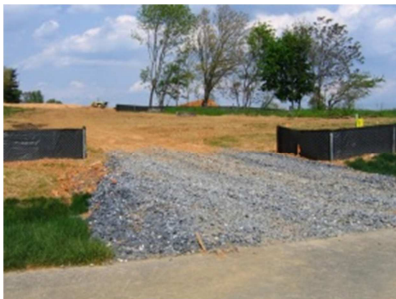
Well maintained site entrance.
