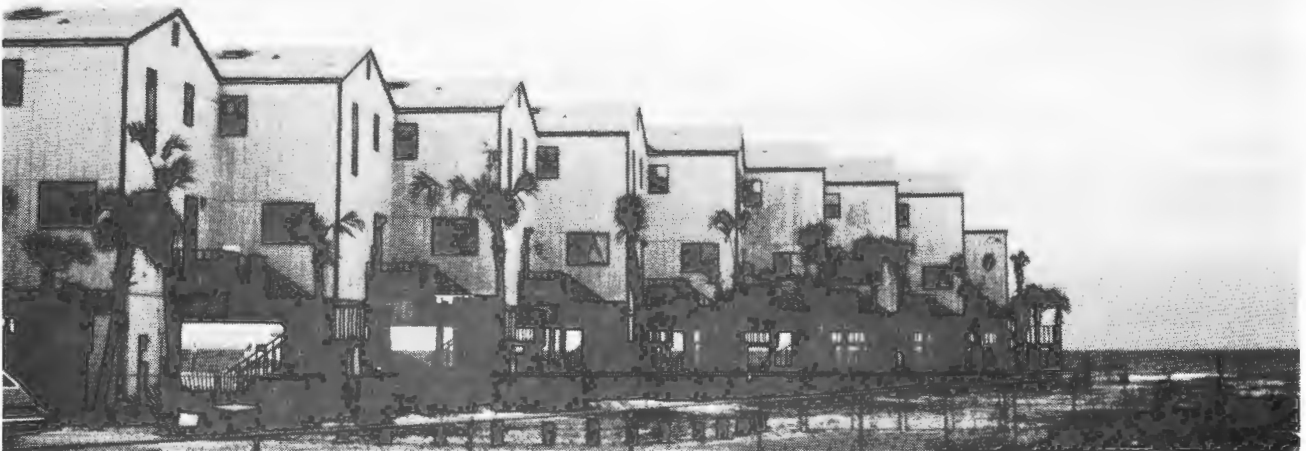
Figure 3.27. This is a good example of how the configuration of a cluster layout can contribute to functional advantage as well as visual appeal. The sawtooth arrangement allows for two sides of each unit to have access/view to the ocean. This form also breaks up the long, continuous (and often monotonous) wall approach, thus adding variety and interest. With this configuration the materials, treatment and form of the units can be simple but still attractive.
