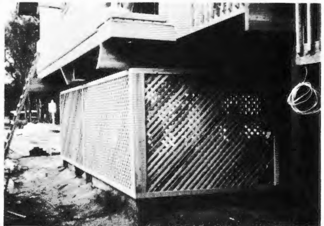
Figure 4.54. Breakaway Walls
