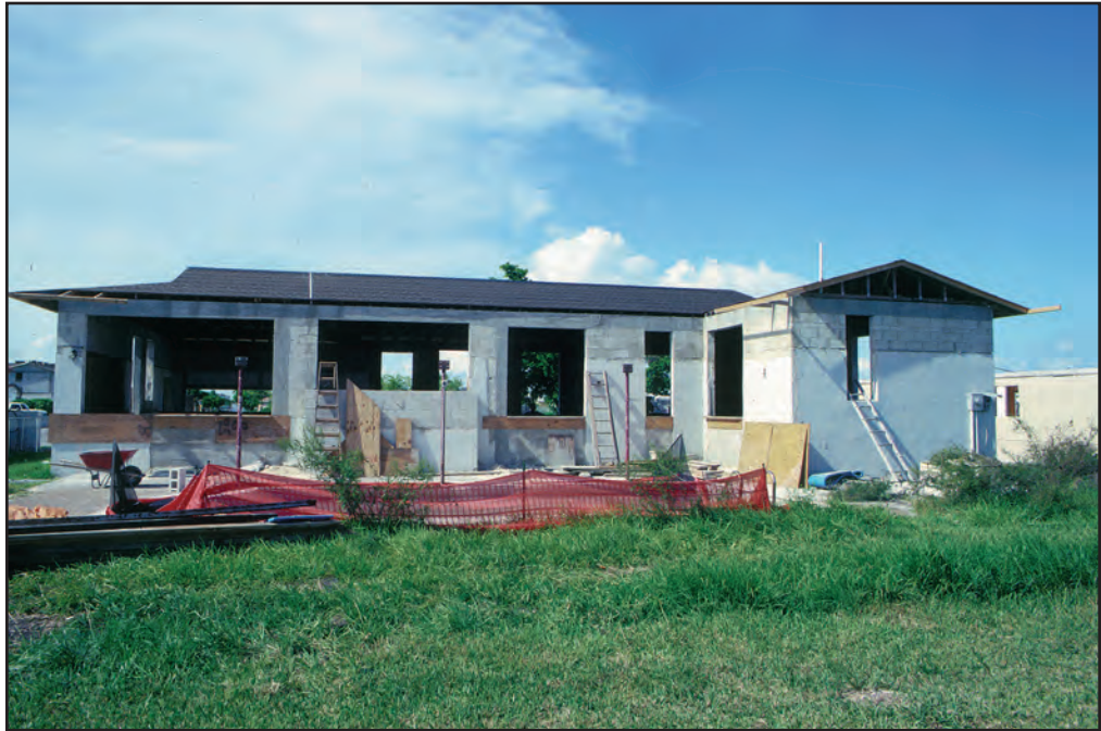
Figure 28 The bottoms of the original window openings are raised with concrete blocks.
