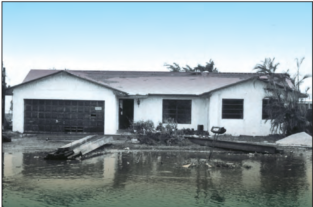
Figure 73 Like the houses shown previously, this one-story house, with its concrete block walls, concrete slab foundation, and attached garage, is typical of the houses in the area affected by Hurricane Andrew.
