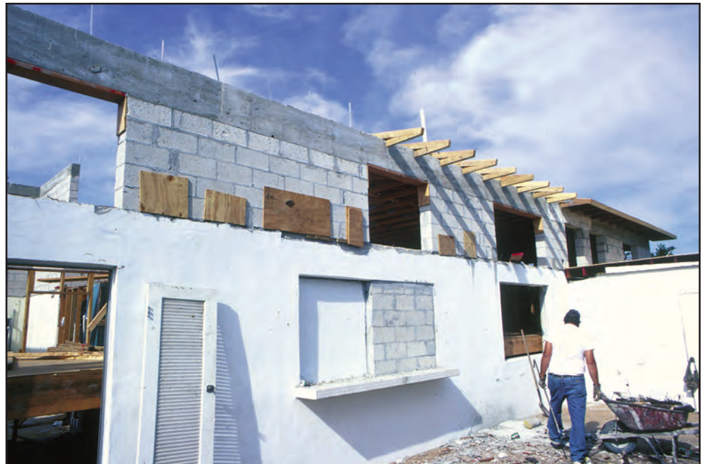
Figure 67 The extended first-story walls.
